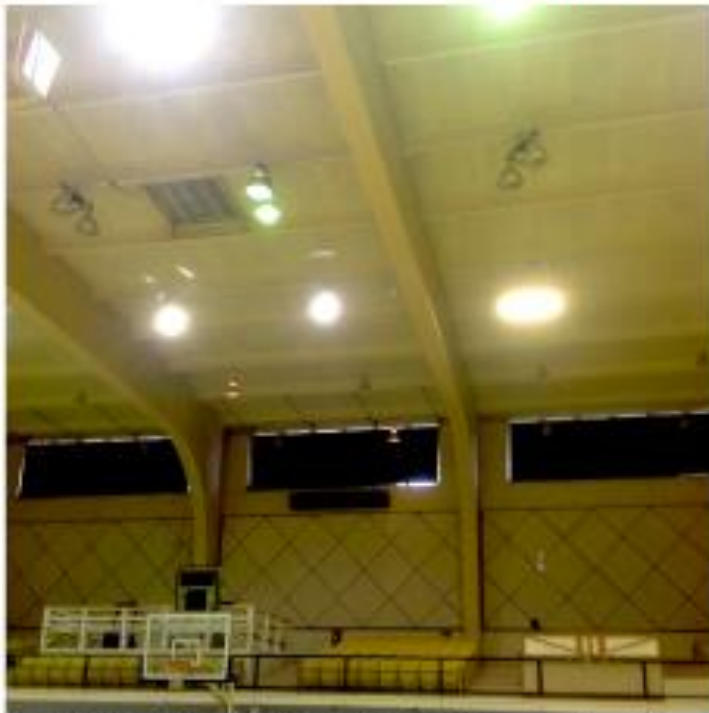
HID lighting (Metal Halide & Mercury Vapor)
