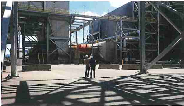
First Energy employees Hank Boka and Doug Colafella inspect the W.H. Sammis power plant in Ohio.
